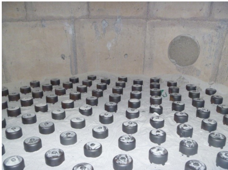
Figure 10. Holding vessel internals.
